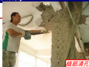
柱梁接頭植筋鑽孔
